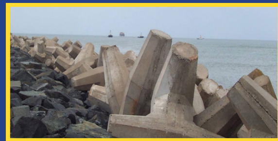
Kolos Casting & Strengthening of South Breakwater Adani Krishnapatnam Port, Nellore
